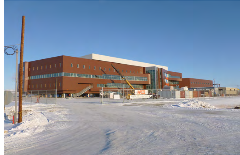
NSHC Regional Hospital (E. Bechtol)
