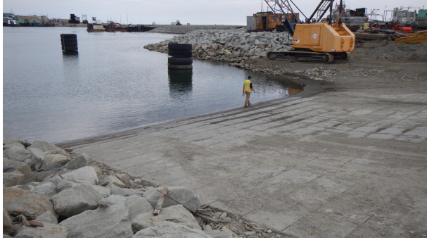
Barge ramp and dolphins from shore
