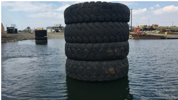
Barge ramp dolphins
