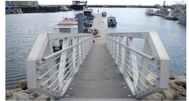
Float and ramp
