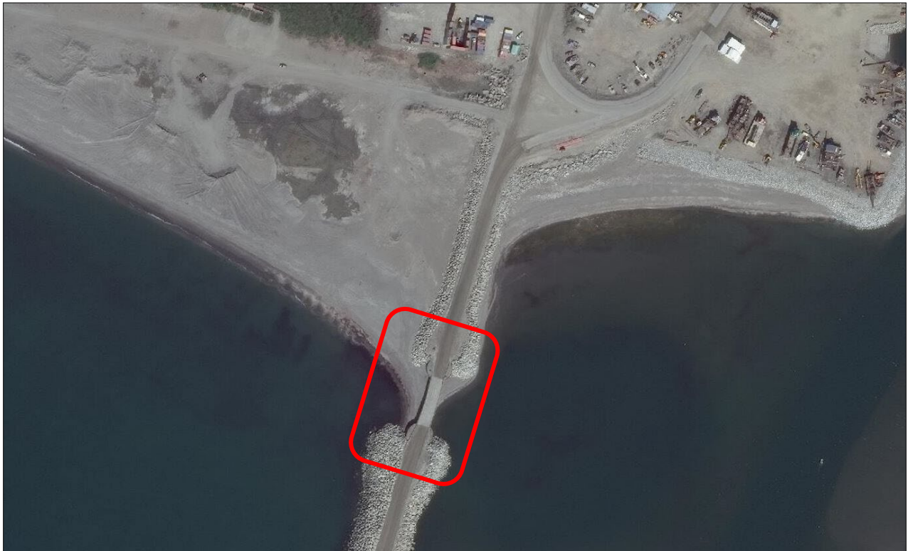
Figure 7. Aerial view of Nome Causeway Breach Bridge in June 2009; Area of Potential Effect outlined in red.
