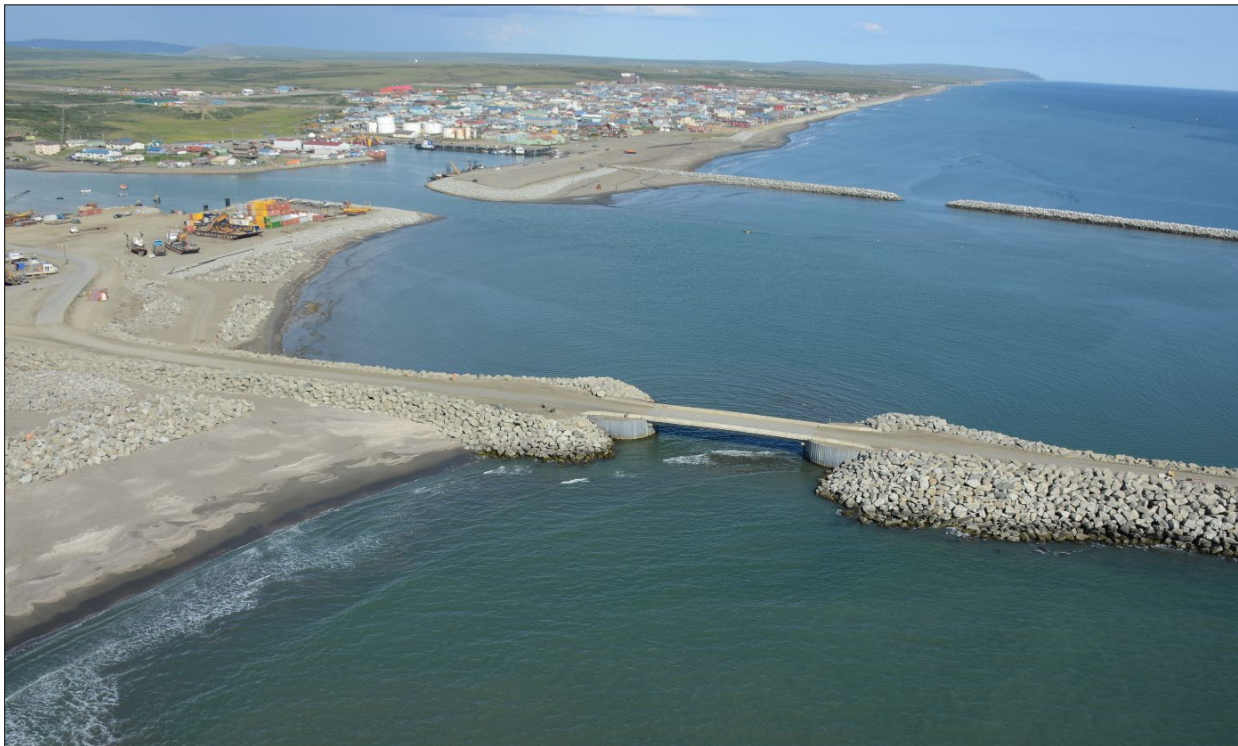
Figure 5. Oblique view of the Nome Causeway Breach Bridge in 2015 (Photo courtesy City of Nome).
