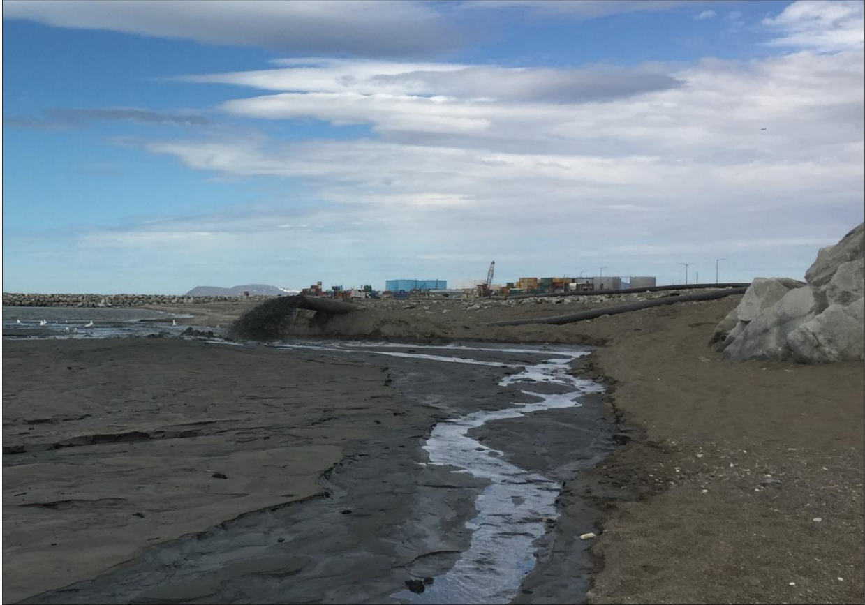
Figure 4. Dredged materials are deposited via temporary pipeline in nearshore waters just east of the eastern breakwater to nourish the beaches in front of town.
