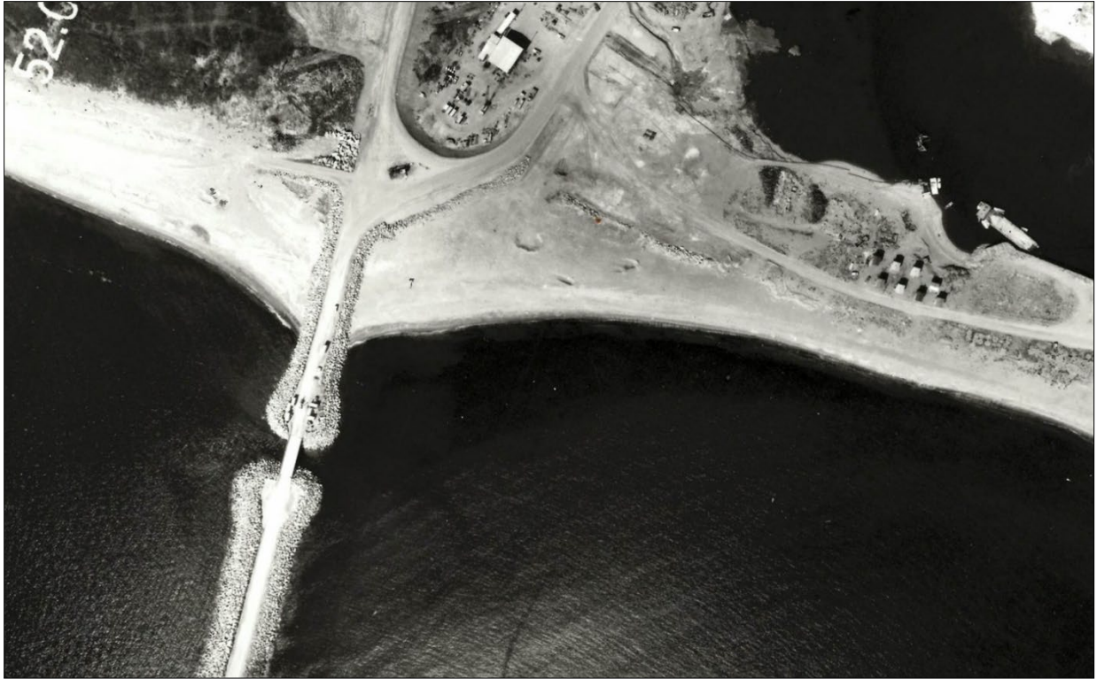
Figure 2. Aerial view of the Nome Causeway Breach Bridge in 1988.
