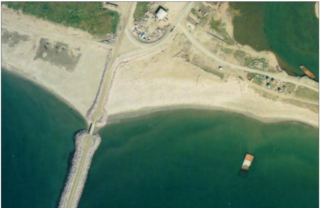
Figure 3. Aerial view of Nome Causeway Breach Bridge in 2003.
