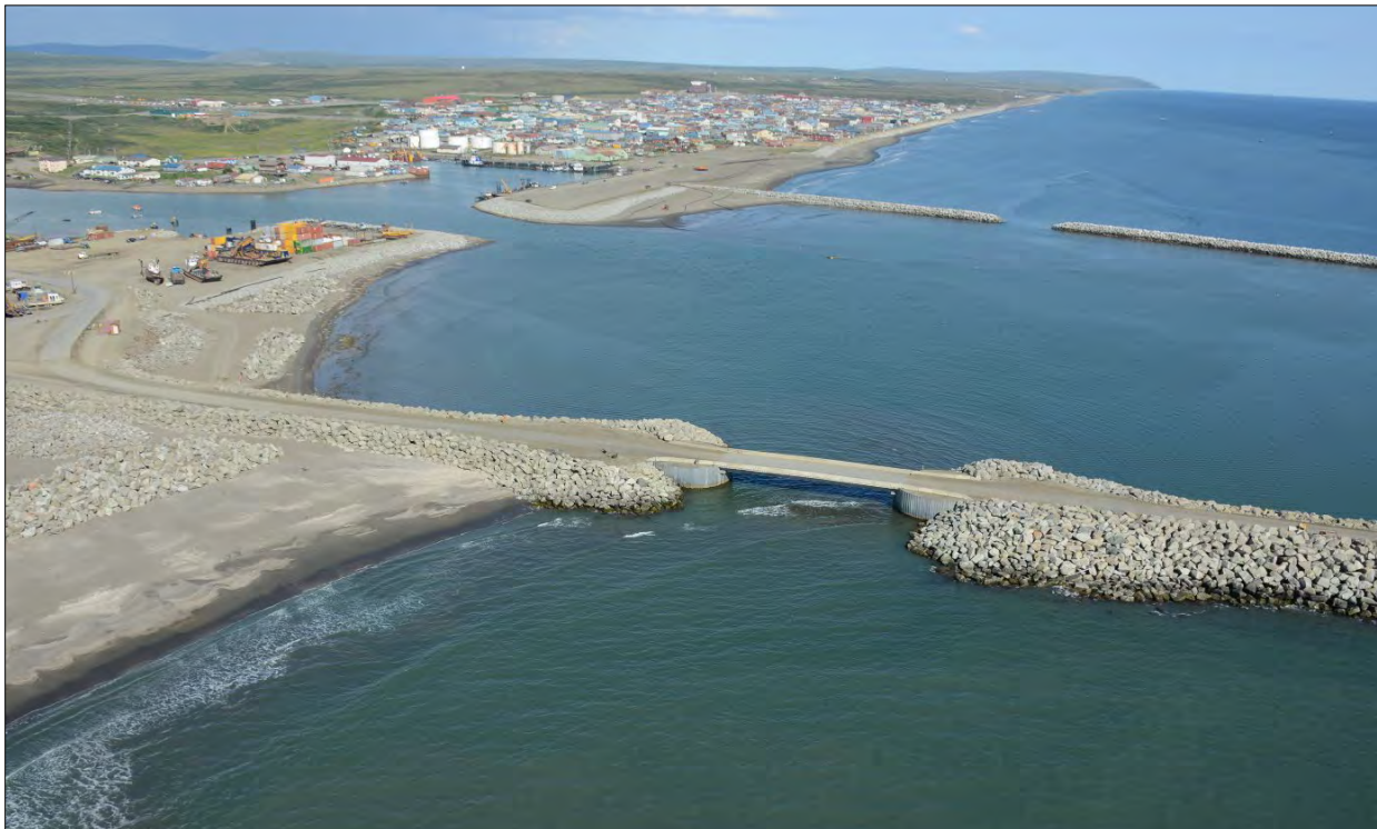
Figure 5. Oblique view of the Nome Causeway Breach Bridge in 2015 (Photo courtesy City of Nome).
