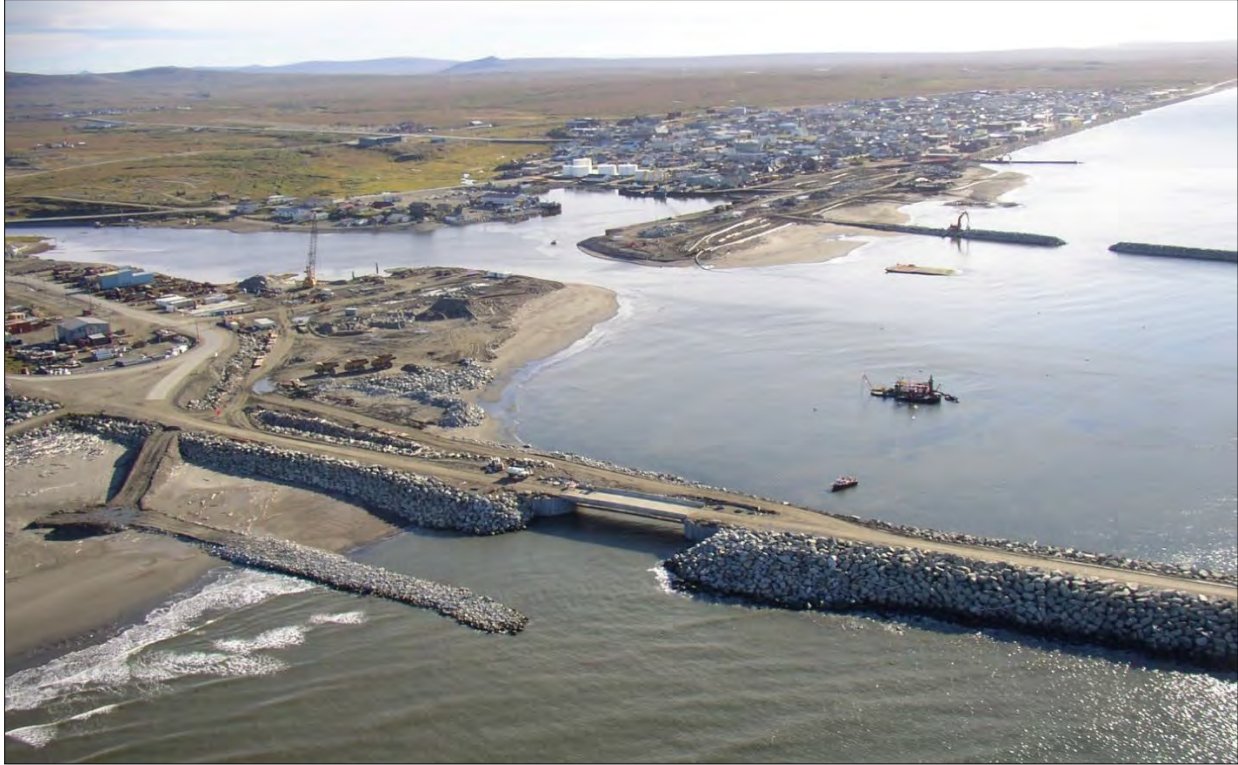
Figure 4. Oblique view of temporary groin and road during bridge reconstruction in 2005 (Photo courtesy of City of Nome).
