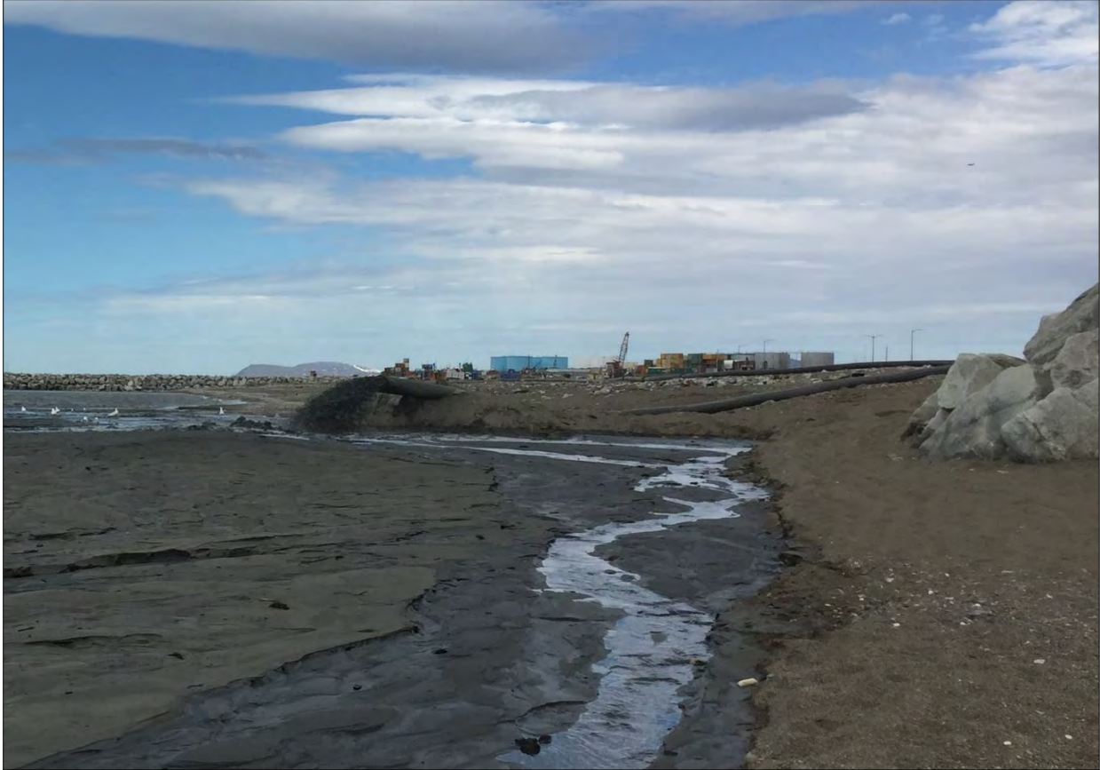
Figure 4. Dredged materials are deposited via temporary pipeline in nearshore waters just east of the eastern breakwater to nourish the beaches in front of town.
